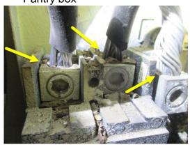
☐ Improper fasteners – Screws for pantry box should have a flat tip, not pointed
