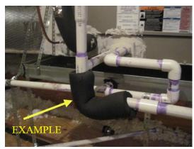
☑ Deficiencies in condensate drain and/or secondary pan and drain lineSecondary drain outlet is plugged
