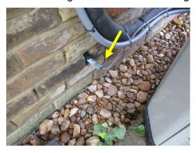
✓ Improper relief line. A smooth copper pipe or CPVC drain line required
